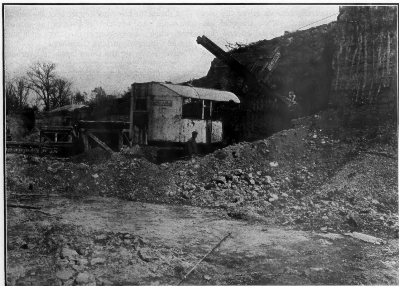
Shovel End of Stripping Operation
